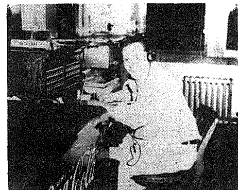
At The Switchboard
