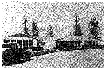
Children's Ward (now college and academy classrooms)
