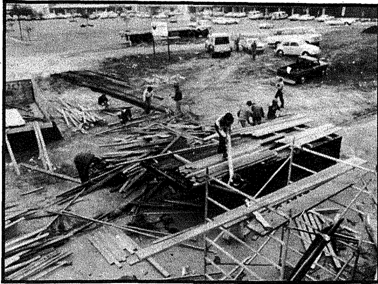
The building parts are coded and then loaded onto trucks.
