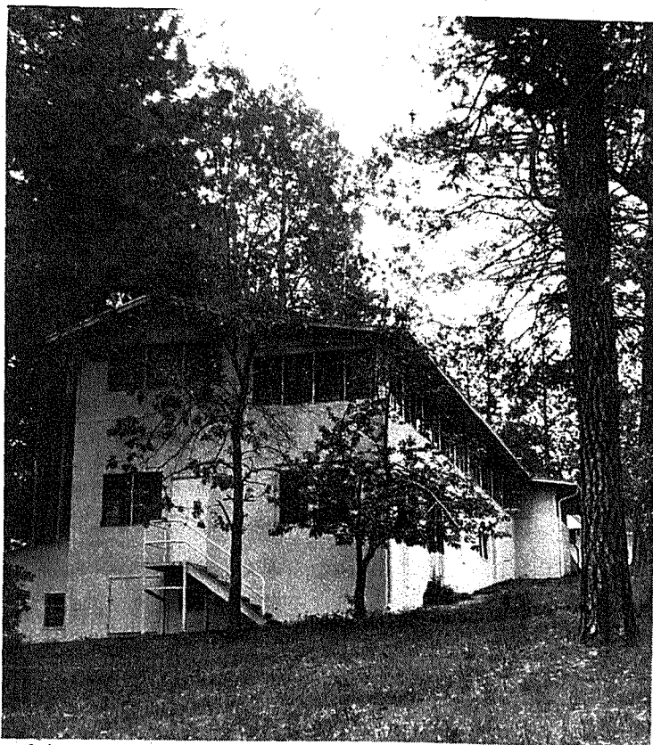
This ward unit, looking through the tops of the trees, is typical of several such buildings on the property.
